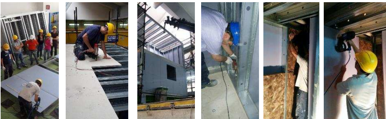
Figure 5. Mounting of structural elements of the mock-up.
