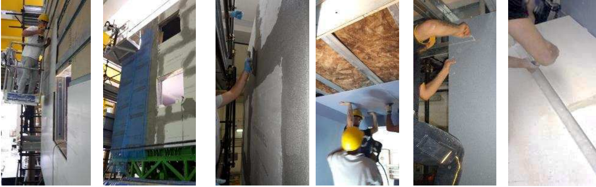
Figure 6. Mounting of finishing products of mock-up
