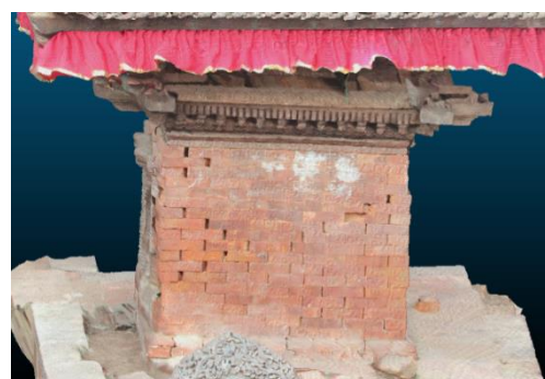
Figure 5. Model of a temple with cracks induced by earthquake.
