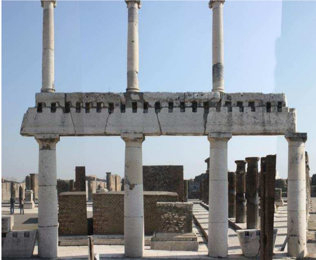
Fig. 1 Two-storey colonnade with multi-drum columns and multi-block segmented trabeations
