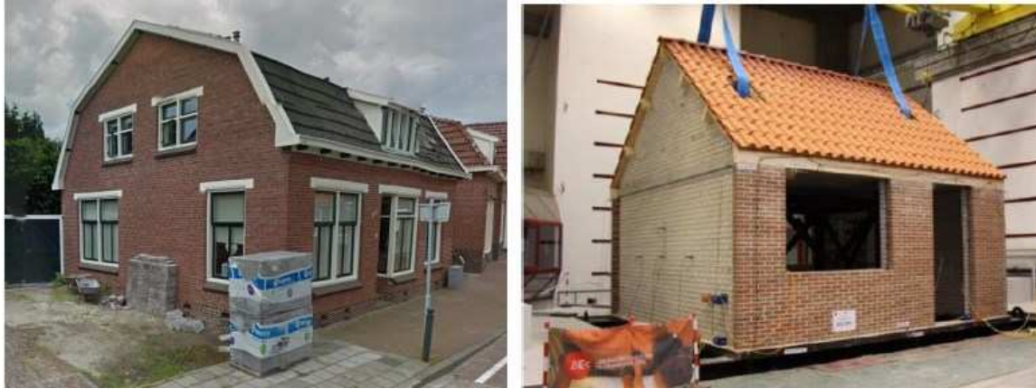
Figure 3. Typology buildings analysed by Mozayk (2017): Nieuwstraat 8 index building (left) and LNEC-BUILD1 (right)
