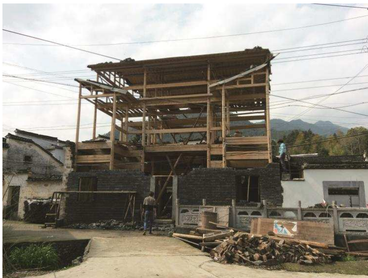
Figure 2. Street view of the carpenter's own house under construction, March 2015.
