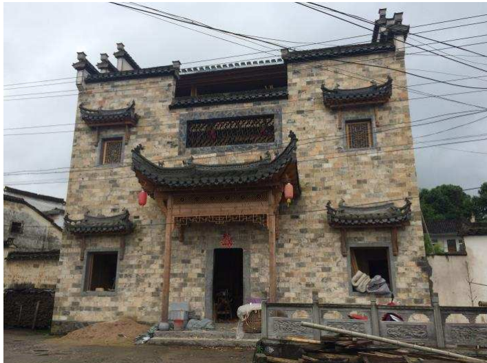
Figure 6. Street view of the carpenter's own house nearly construction, July 2016.
