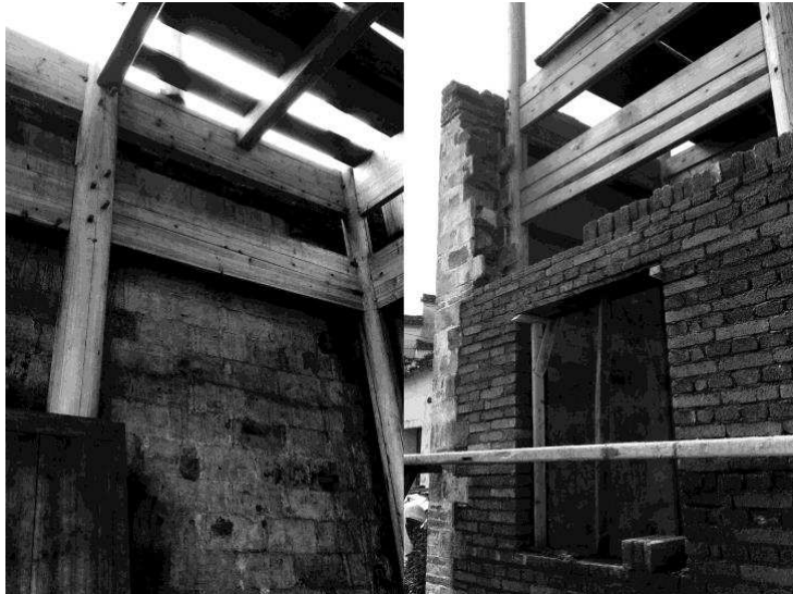
Figure 4. Working with the given site condition and available materials: new timber structure supports the existing loadbearing wall (left); new brick freestanding wall works with the existing wall (right).
