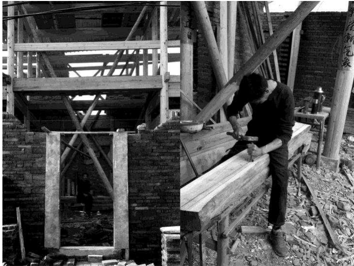
Figure 3. Almost a one-man-practice without any drawing: the carpenter sitting in the construction site of central hall (left); His ongoing beam work of mortise and tenon for upper bedrooms (right).
