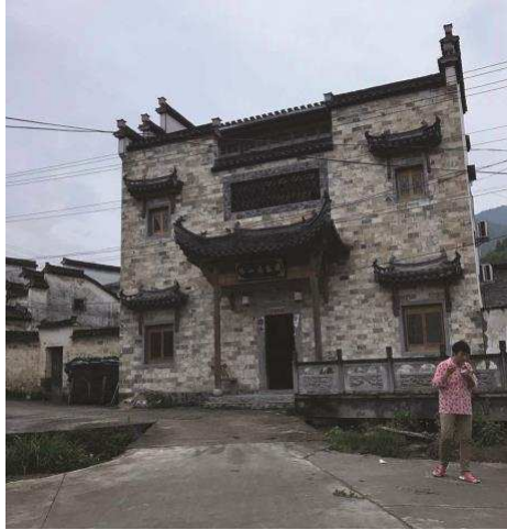
Figure 7. Street view of the carpenter's own house in use, August 2017.
