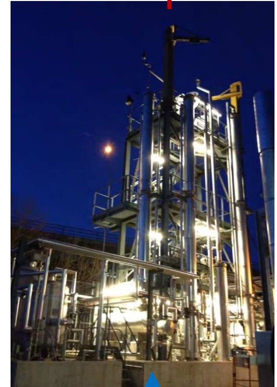
Carbon Capture Plant
