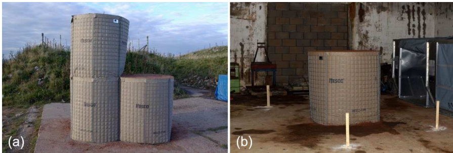
Figure 4. Gabions after filling (a) exterior gabions P1-P3 and (b) interior gabion I1.
