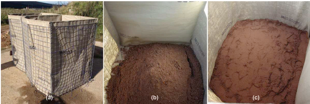
Figure 3. Gabion filling method: (a) deployment, (b) addition of fill material layer and (c) distribution and compaction of layer.
