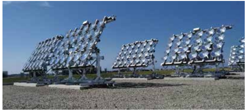
▲ This tracking concentrator type solar array , which is in field testing by Actree Co. Ltd. in Ishikawa Prefecture, Japan, automatically follows the sun across the sky.
