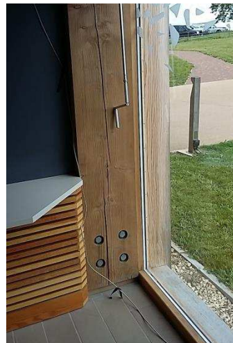
Figure 6 Vertical cracks occur in a column
