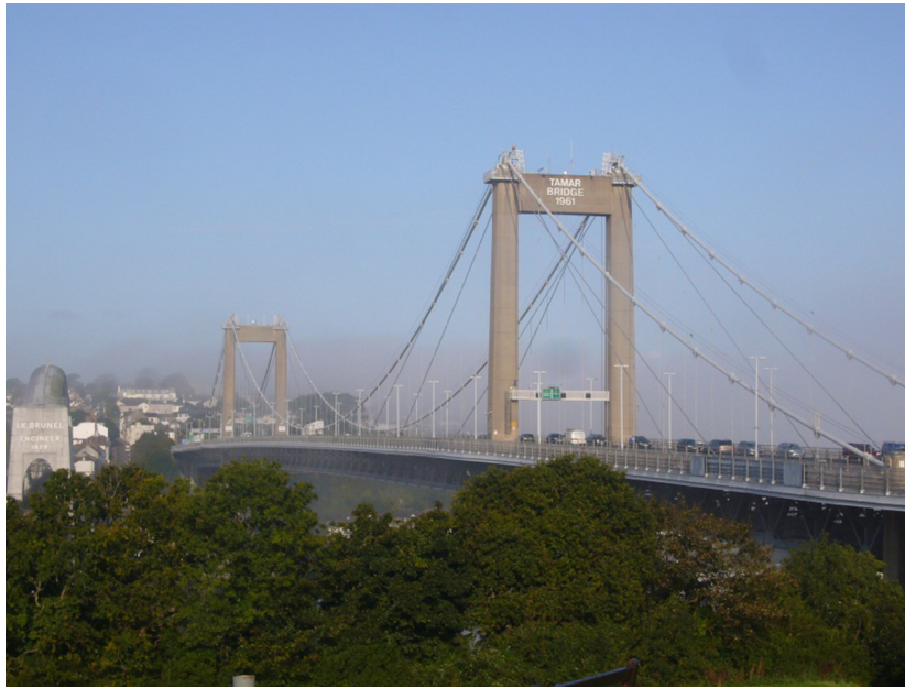
Fig. 1. The Tamar Suspension Bridge.
