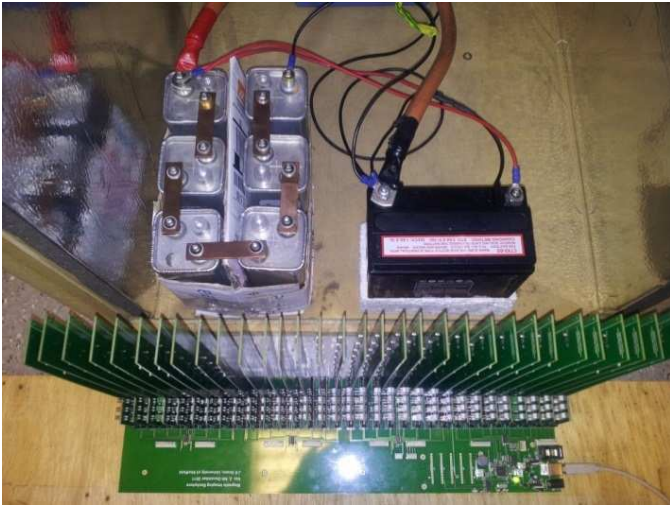
Fig. 10. left: Ultracapacitor bank. right: AGM Battery (on a 50 mm polystyrene block). Details given in Section VII.
