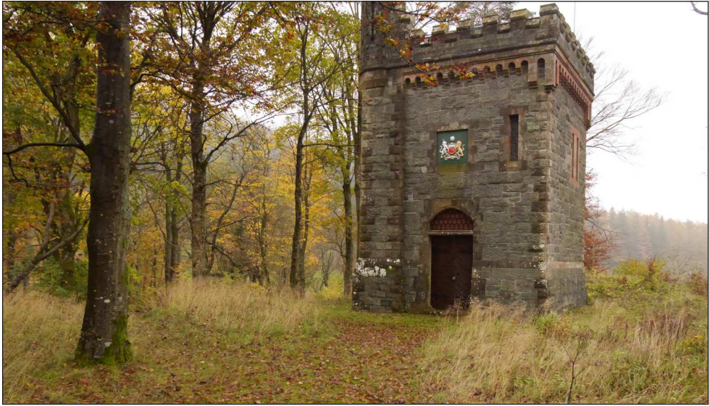
Figure 1: The pump house of Thirlmere reservoir in the Lake District hides its intervention in the landscape behind heritage tropes. Concepts of ‘forever’ overlap with ‘timeless nature’ (Photo Sarah May).
