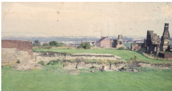
Fig. 5 – Photograph of the west range of buildings taken in 1969 (looking east)
