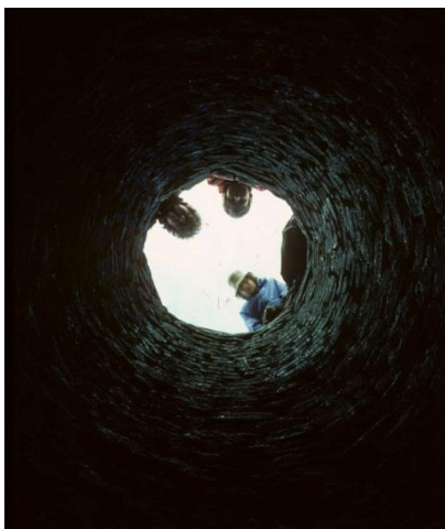
Fig. 40 – Looking down the well found near to the south end of the long gallery
