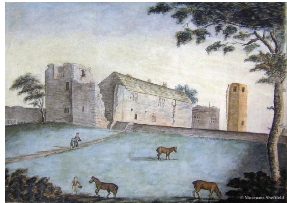
Fig. 6 – Watercolour of the long gallery and surviving tower by David Martin (1795)
