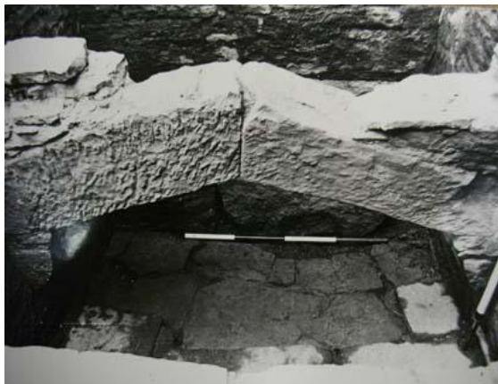
Fig. 22 – The garderobe in the ‘Wolsey Tower’; this was in the room on the far side in fig. 21
