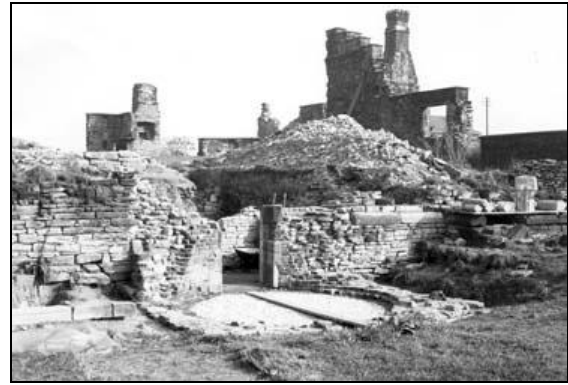
Fig. 13 – Excavation of the rooms behind Tower A in 1970
