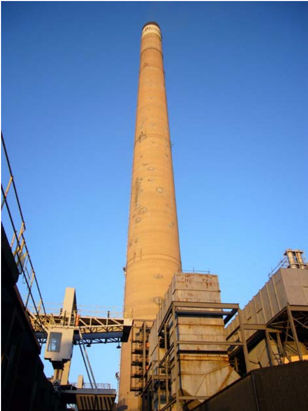
Figure 1 Chimney at Rugeley Power station
