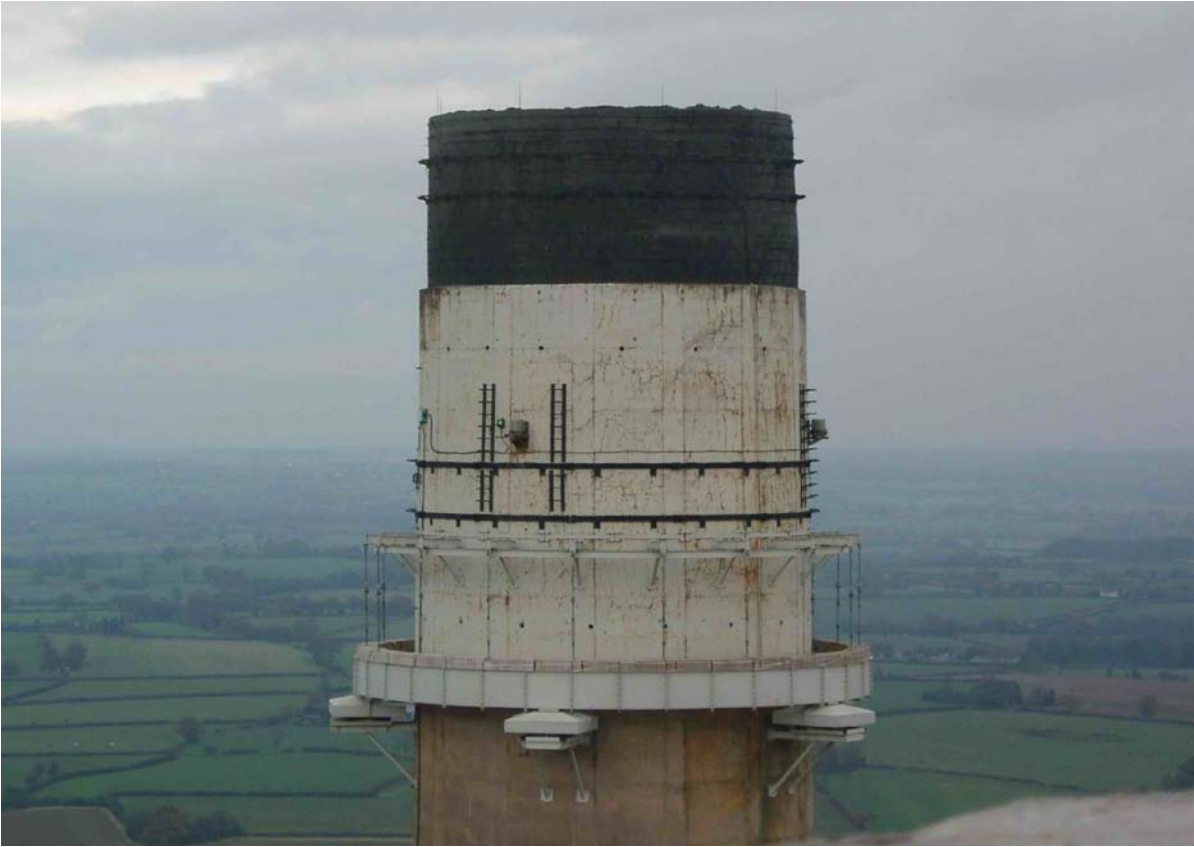
Figure 7 View from new chimney showing TMD supports, mass ring and dampers
