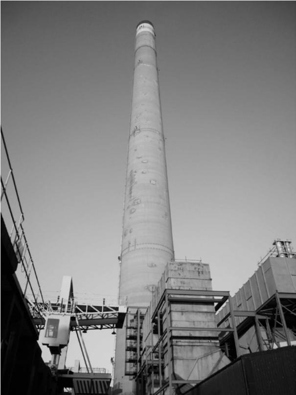
Figure 1 Chimney at Rugeley Power station
