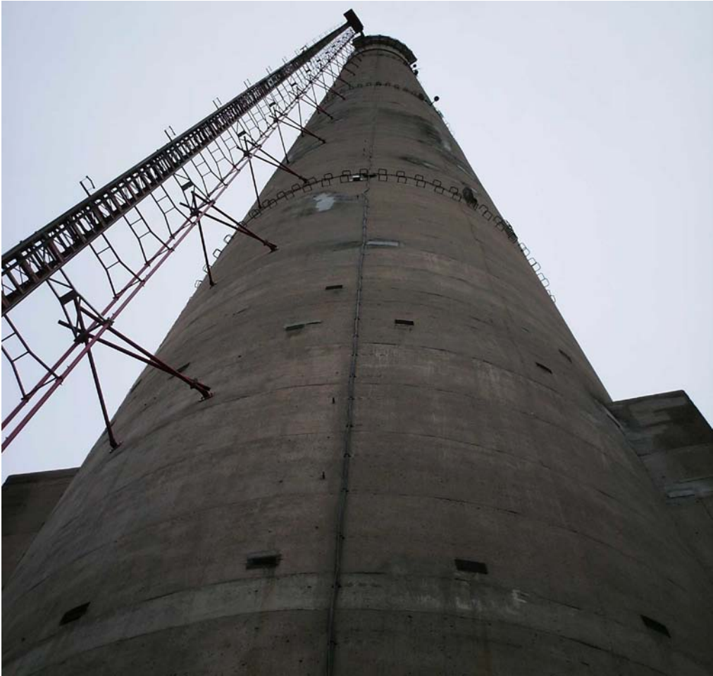
Figure 5 TMD under construction, with lower accelerometer box in position and flue openings flanking chimney
