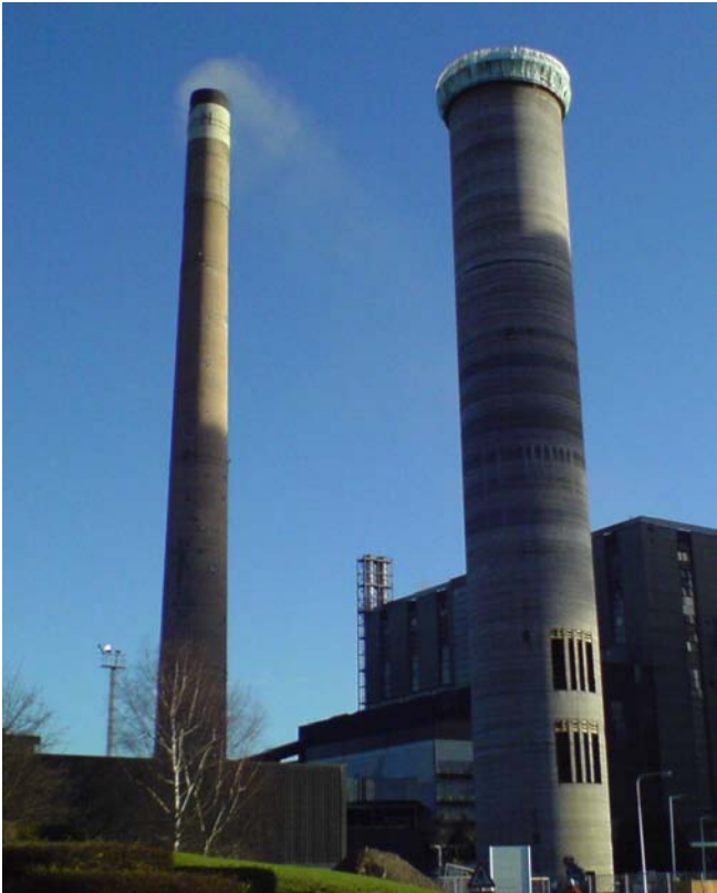
Figure 2 New Chimney under construction
