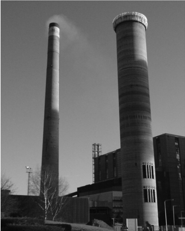
Figure 2 New Chimney under construction
