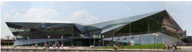
Figure 1. The Crystal building in East London.
