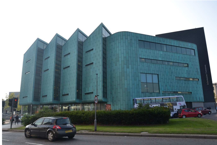
Fig. 9. External view of the Information Commons.
