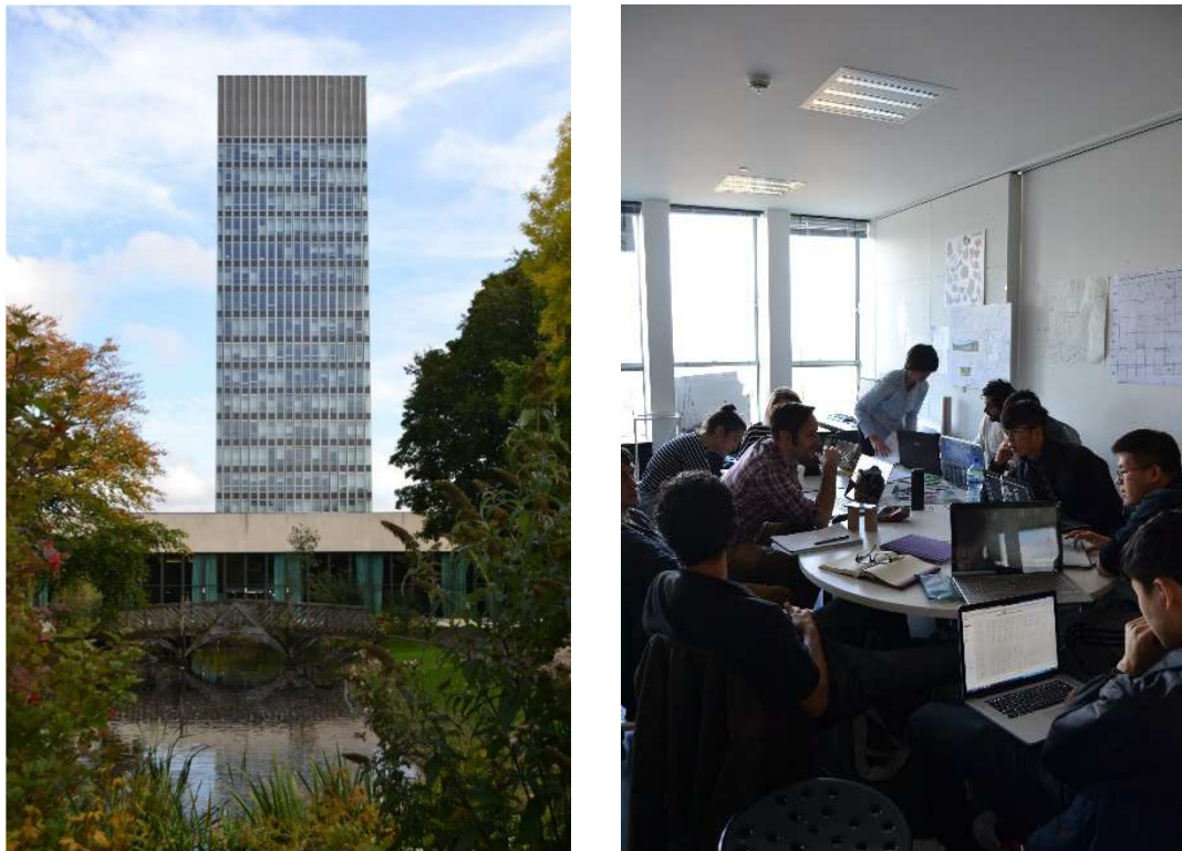
Fig. 1. The Arts Tower exterior and internal study space.
