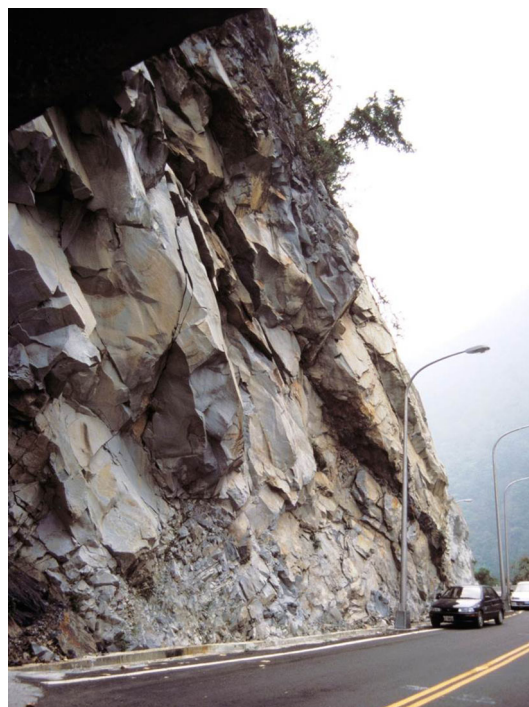
Fig. 1 Slope with daylighting rock slabs threatening highway in central Taiwan. The incipient nature of the discontinuities contributes tensile and shear strength and allows temporary stability
