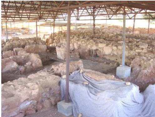
Figure 1: A temporary structure becoming permanent in Sapinuwa, Ortaköy, Turkey (Ertosun [3])
